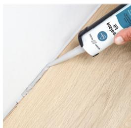
**Step 2:** Apply the **Hydro+ Sealant kit** on top of the Fillertwine. The Sealant kit should touch the wall and the laminate and be applied in a way that it completely closes the gap. With floor profiles, use sealant on top of the Fillertwine before you install the profile to avoid water contact with the side and the base of the laminate.
